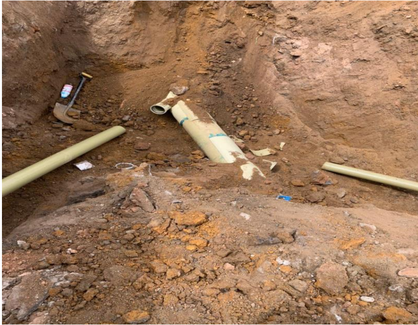
Pipe laying in progress
