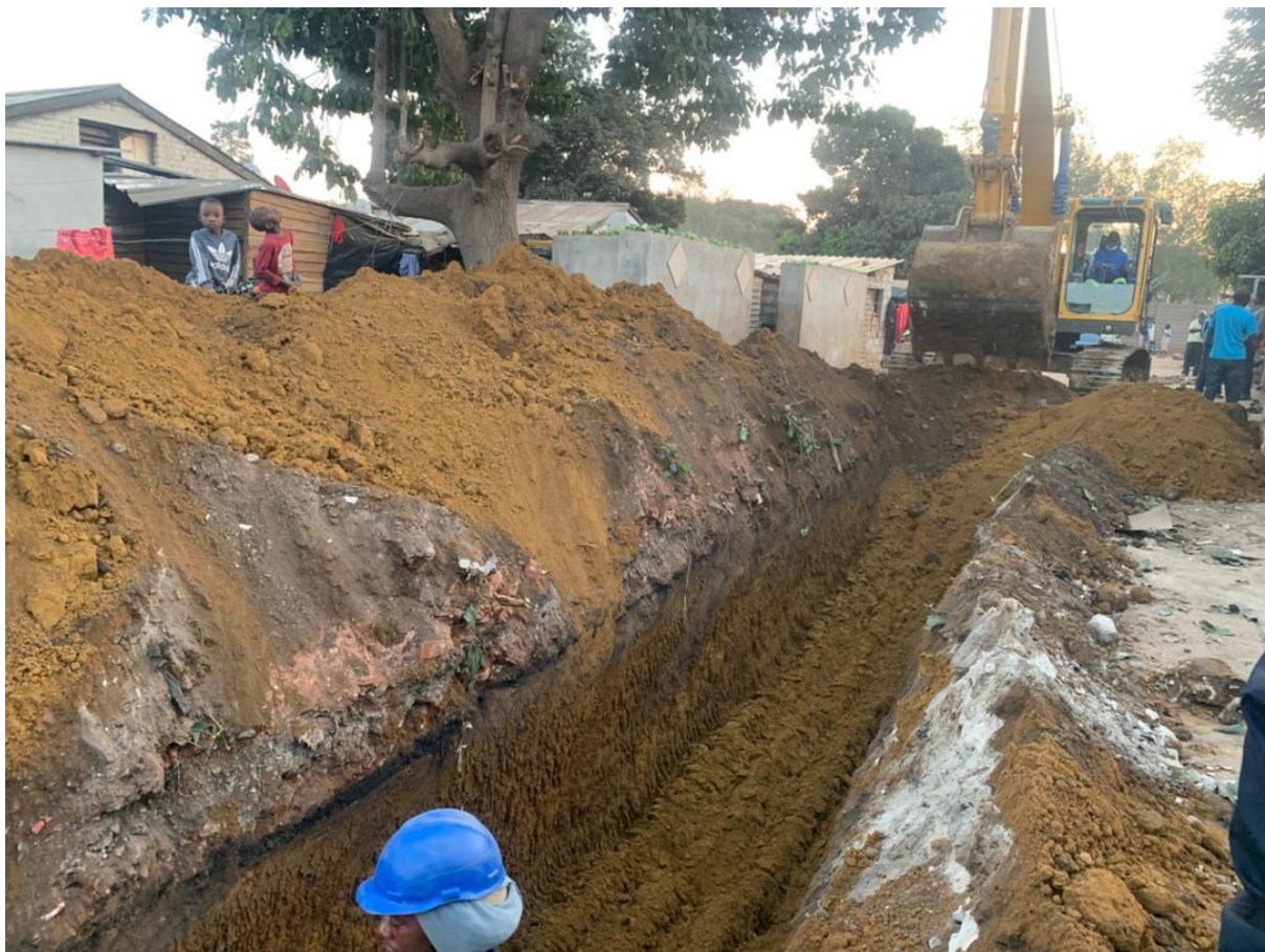
Newly acquired excavator at work in Mbare
