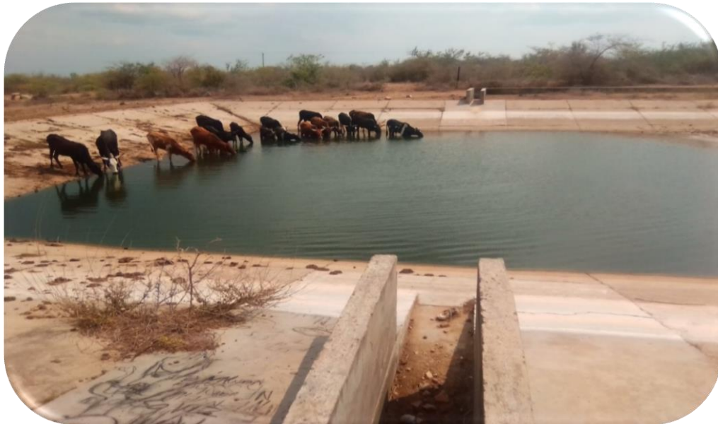
Picture by Auditor: Kotwa Sewer Ponds
