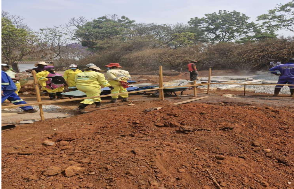
Construction of Marlborough Clinic
