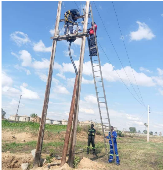
1Installation of power cables for Firle Units 5A and B
